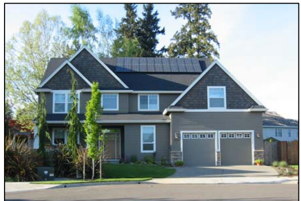
2.9 kW solar electric system in Beaverton
