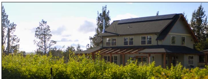
2.3 kW solar electric system in Redmond
