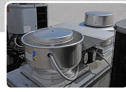
To address the air particulate matter and reduce build-up in ducts, Multi-Services, Inc., selected replacement bath and dryer exhaust fans. They also added new pressure controls to the dryer shafts to monitor when a dryer turns on, increasing fan speed when necessary. The new rooftop exhaust fans are variable-speed, energy-efficient models equipped with speed and constant pressure controls, helping to reduce energy costs and increase tenant safety.
