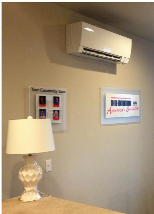
The second story ducted DHP is shown in Figure 3 (left image). There are vents above the DHP unit leading to the internal ducting. Although uncommon, at this particular site there are also vents above the door (right image) to draw air from the area directly outside the room where the DHP indoor unit is located. A programmable thermostat that is located in a utility room controls the indoor units. The occupants cell phone is used to control the thermostat.
