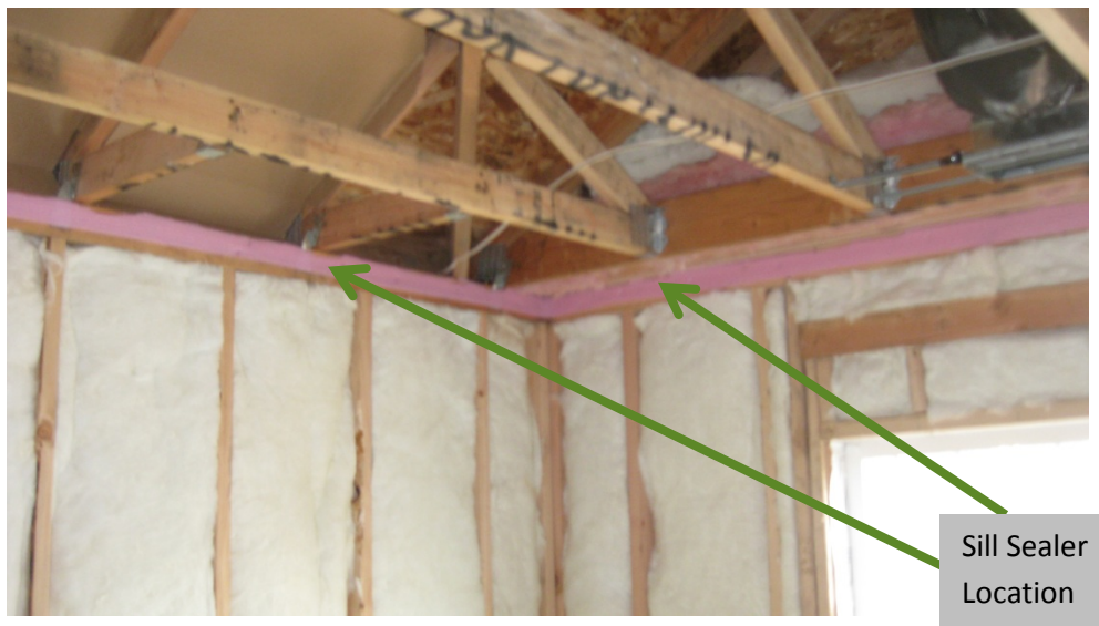
Figure 1 – Sill Sealer Gasket Location
