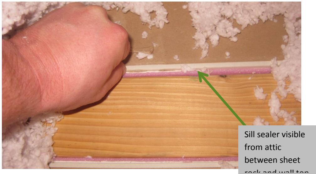
Figure 2 – Sill Sealer Installation confirms from attic
