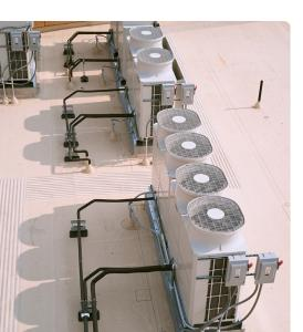
"We went with a system called VRF, which is variable refrigerant flow. This system is unique because it uses liquid to transfer heating and cooling rather than air. So it's much more efficient," said Neil Piispanen, architect and project manager.
