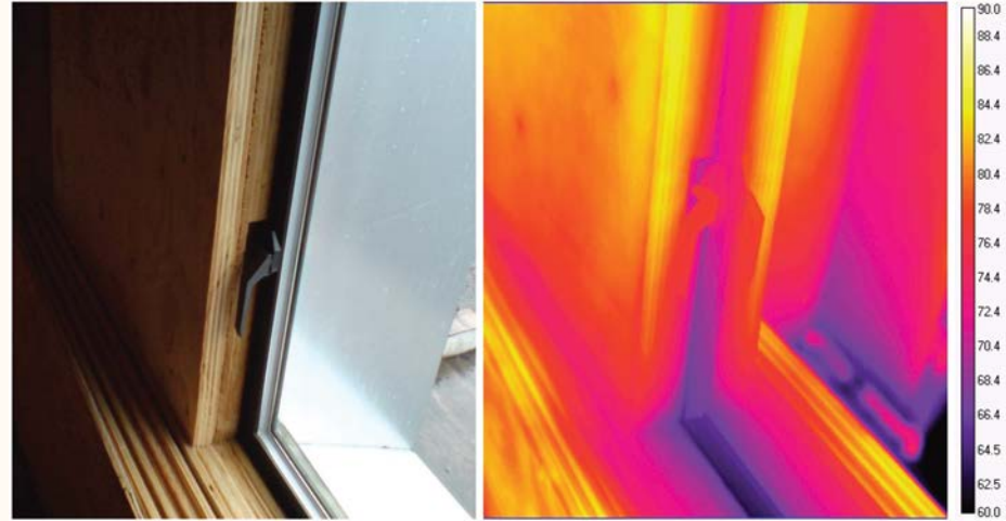
INTERIOR THERMAL IMAGING OF ENCLOSED AND HEATED MOCK-UP; OPERABLE WINDOW
