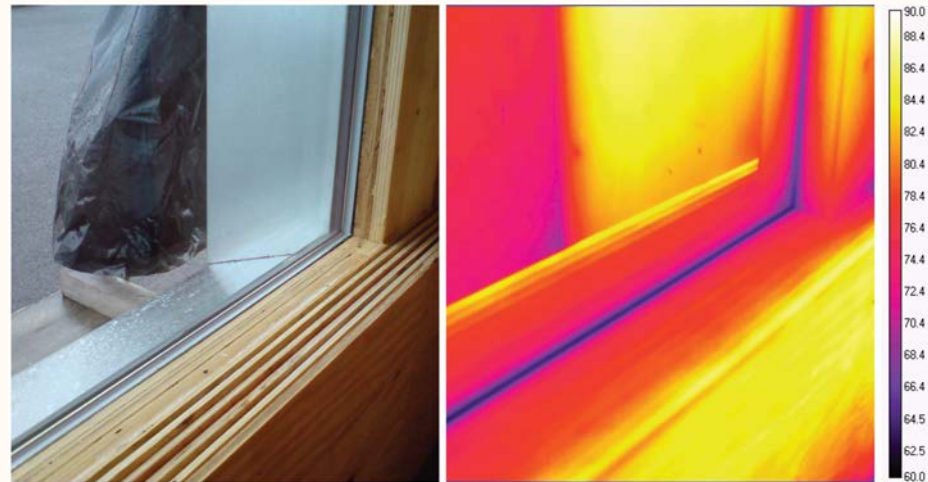
INTERIOR THERMAL IMAGING OF ENCLOSED AND HEATED MOCK-UP; FIXED WINDOW
