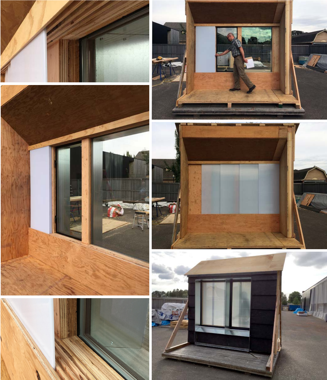
Figure 20: Completed MPP mock-up photos including polycarbonate energy shutter
