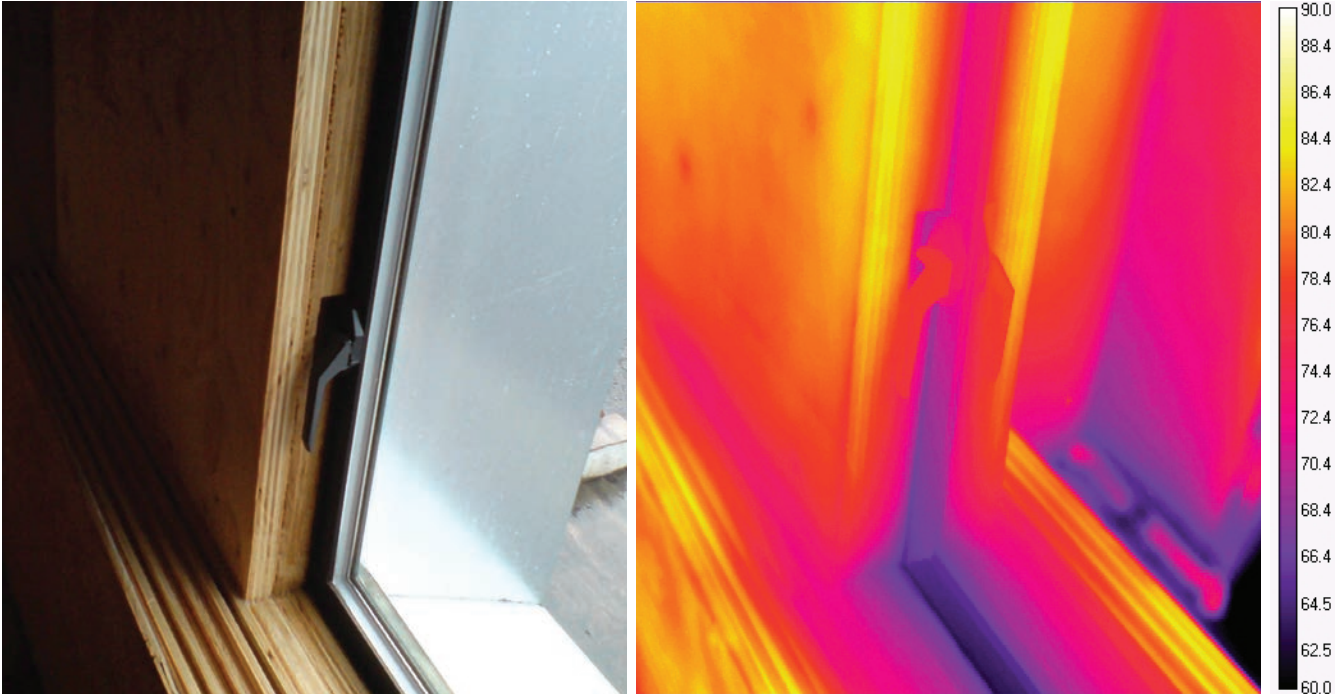
Figure 22: Interior thermal imaging of enclosed and heated mock-up; operable window
