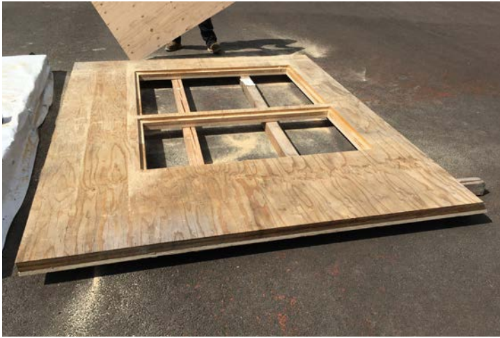
Figure 18: MPP window mock-up construction process photos
