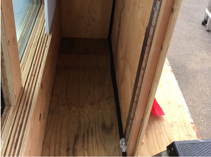
Figure 24: Blower door testing and pressurized smoke testing photos
