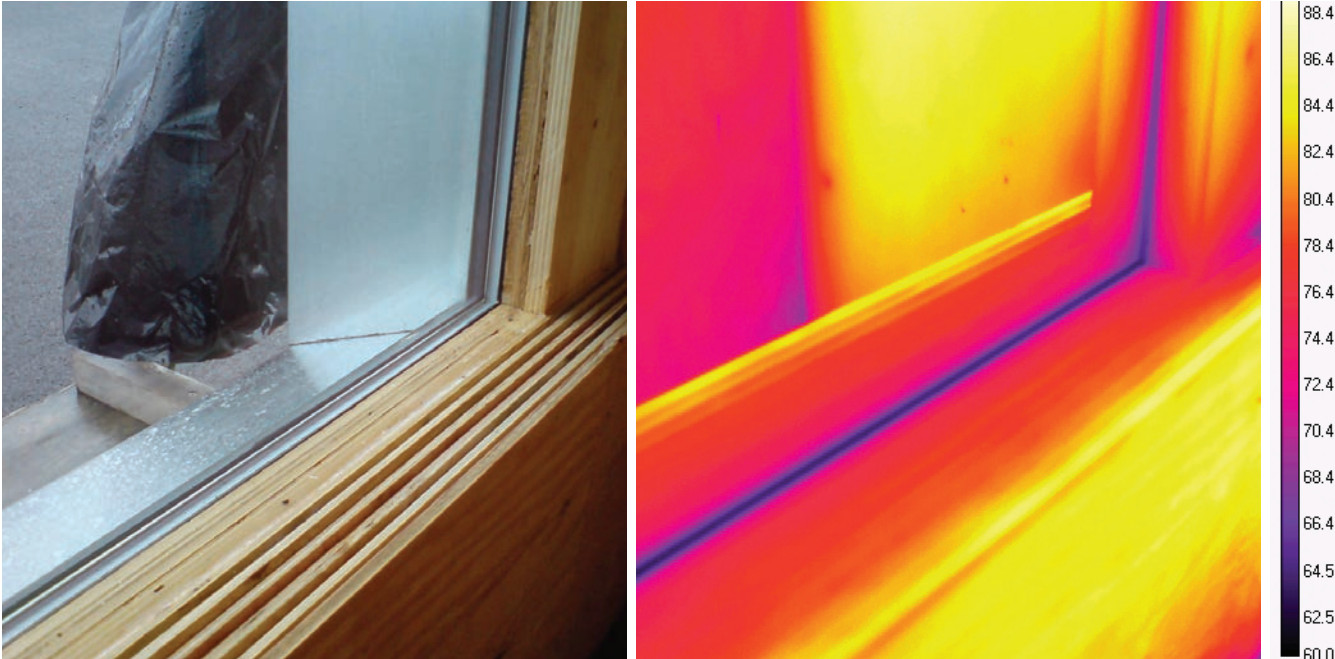
Figure 23: Interior thermal imaging of enclosed and heated mock-up; fixed window
